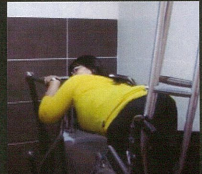
Grab bar in the wrong place
